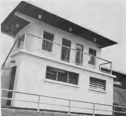
TOP DECK of the new Marine Department facility is slightly reminiscent of a tanker's bridge. The overhang offers protection from sun and rain.
